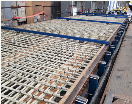
REINFORCING FRP REBAR
