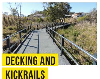
During the process of making the decking and the kickrails, Wagners suppliers use a process of injecting the requested color into its resins to ensure that no edge is left without its color after trimming.
