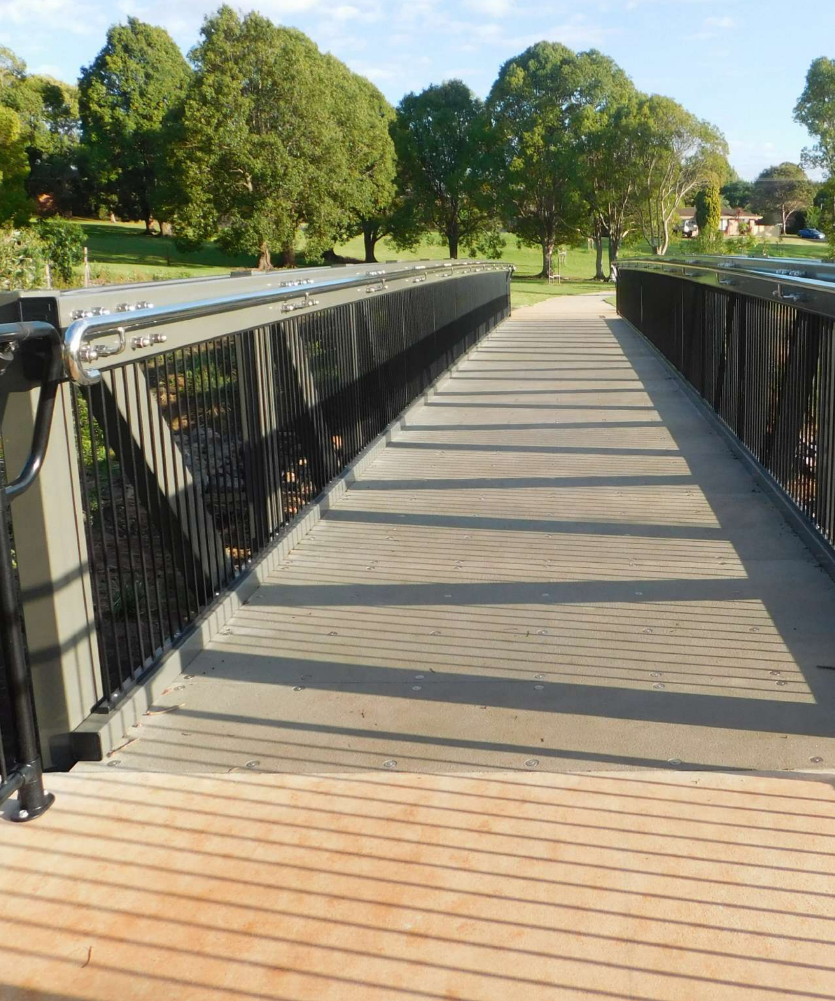
BALLIN DRIVE PEDESTRIAN BRIDGE, TOOWOOMBA, QLD, AU
