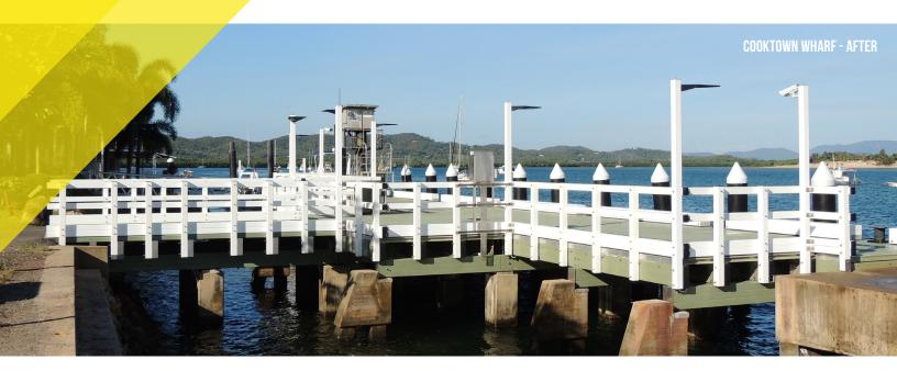
At times, rehabilitation rather than complete replacement of an asset is more appropriate. To ensure safety and longevity of a rehabilitated asset, Wagners have developed a timber replacement system. The system can either replace damaged and deteriorated timber components or provide a complete overhaul of the whole structure.
