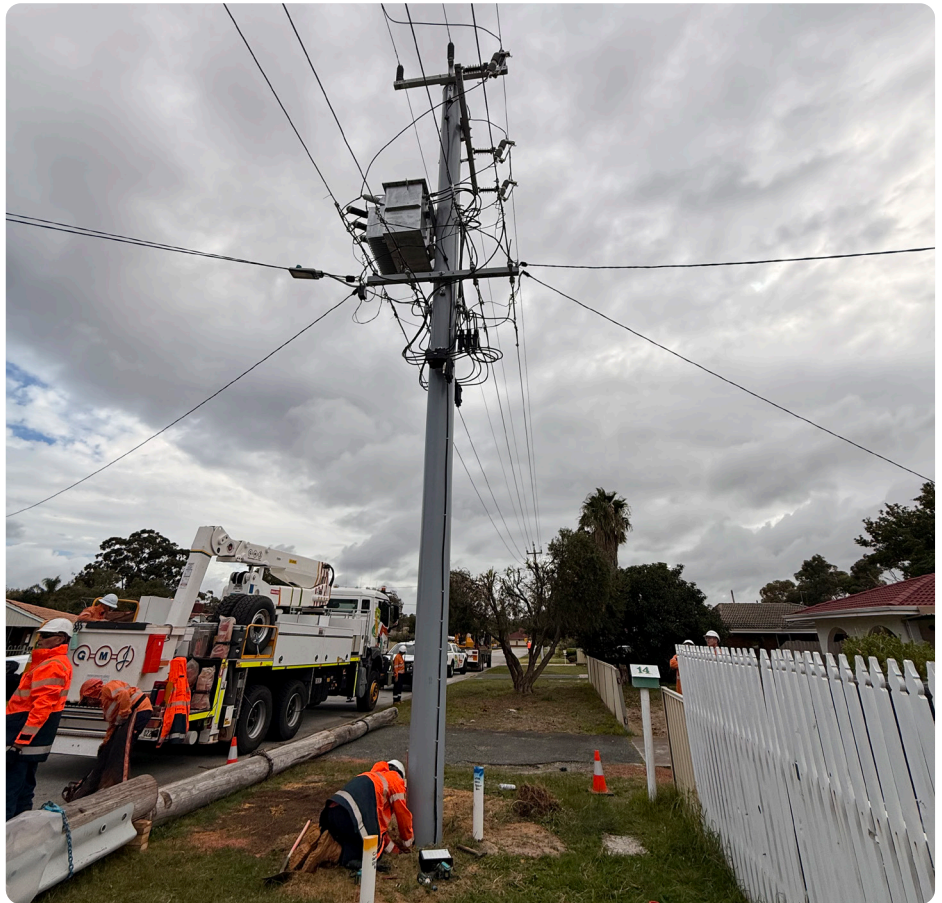
Figure 11 – Installed Wagners pole
