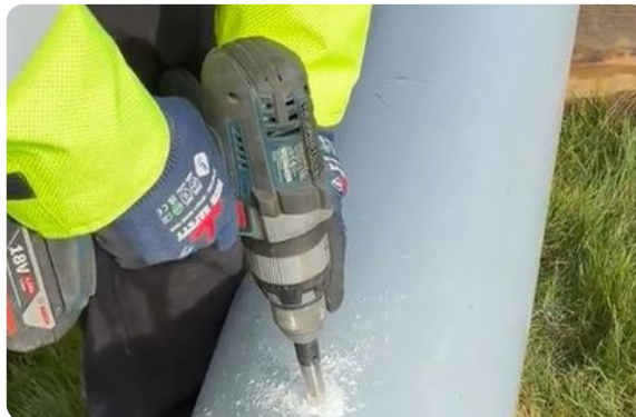
Figure 3 – Drilling a composite pole
